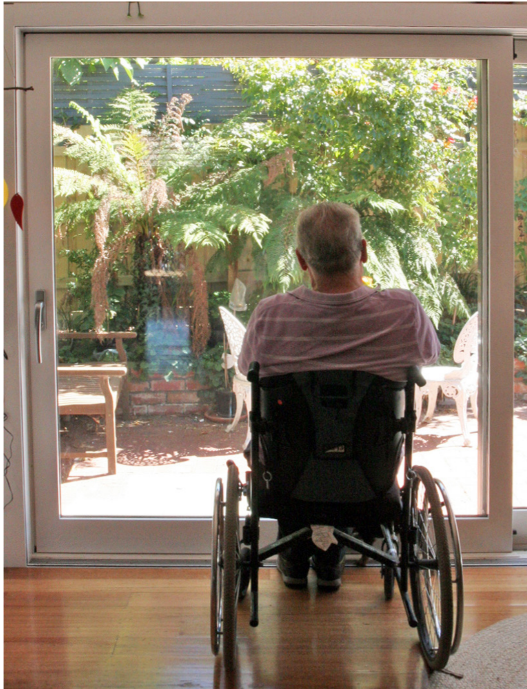
Far right height of sill and proportions of windows has an impact on wheelchair users
