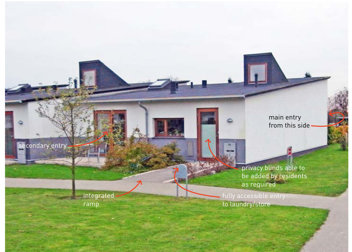
Above Here to Eternity: glass doors are used in place of windows to increase access without compromising on natural light
