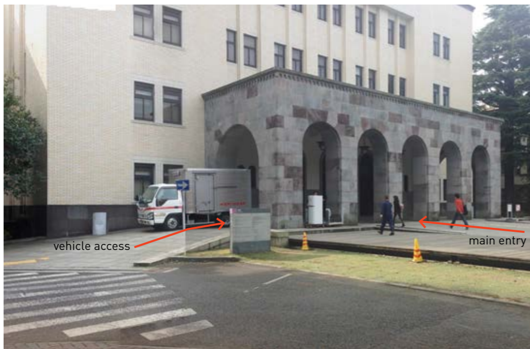
Top Tokyo Institute of Technology: stair entry replaced with deck that ramps up and is flush with the entry
