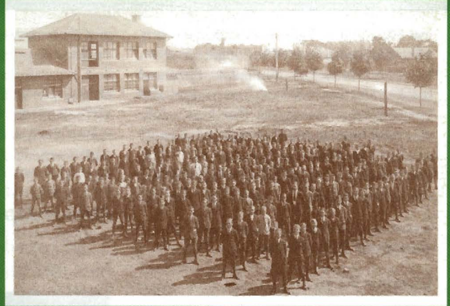
Caulfield Technical School, 1922.
