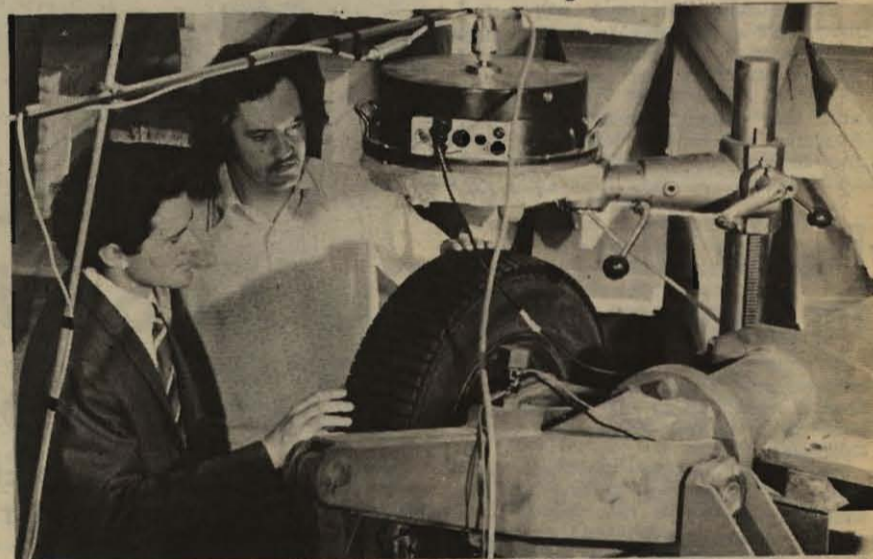
Dr. Alfredson and Stephen Samuels inspect the tyre research equipment in the University's anechoic chamber. The wedge-shaped material in the background absorbs noise.
