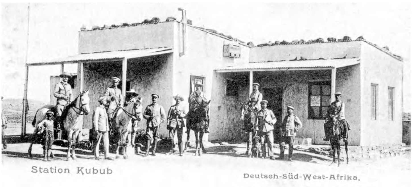
Fig. 116. Kubub Post Office and an Ox Wagon rest point.
