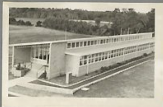
Administrative Block from the Hostel
