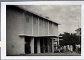
Side view of memorial church.
