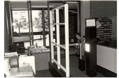
Chisholm-Frankston Library c1980 (Building A)
